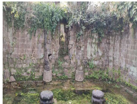
Fig. 3. Recesses in the temple wall.
